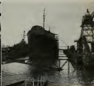
Ship is now in position above blocks and dock will be raised to land her on foundation blocks.
